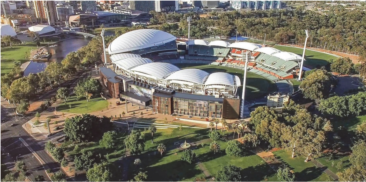
Figure 3.4: Adelaide Oval Hotel integration with stadium
